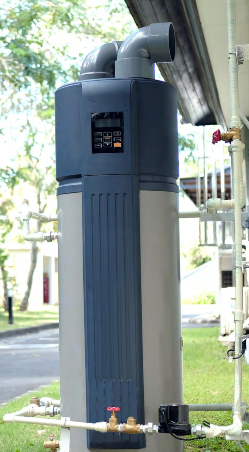
As part of our energy-saving pledge, we have integrated heat pump technology for water heating. This innovative system utilises renewable energy sources, capturing ambient warmth from the air and efficiently converting it into heated water which is then channeled to the resort's facilities.
